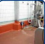
Specialist Contractors, Rüdiger Schmidt GmbH, were asked for advice and they proposed a complete floor repair and high build coating solution, using a VIP 2-component, hot-spray applied, polyurea resin system. This VIP polyurea system is used for highly abrasion and chemically resistant floors, including the incorporation of ballotini glass beads to achieve the level of anti-slip resistance (Class R11), which defines that the surface is suitable for wet food process environments.
